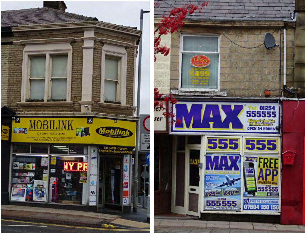
Above – overly large fascia boards/signage - bad practice (unacceptable)
