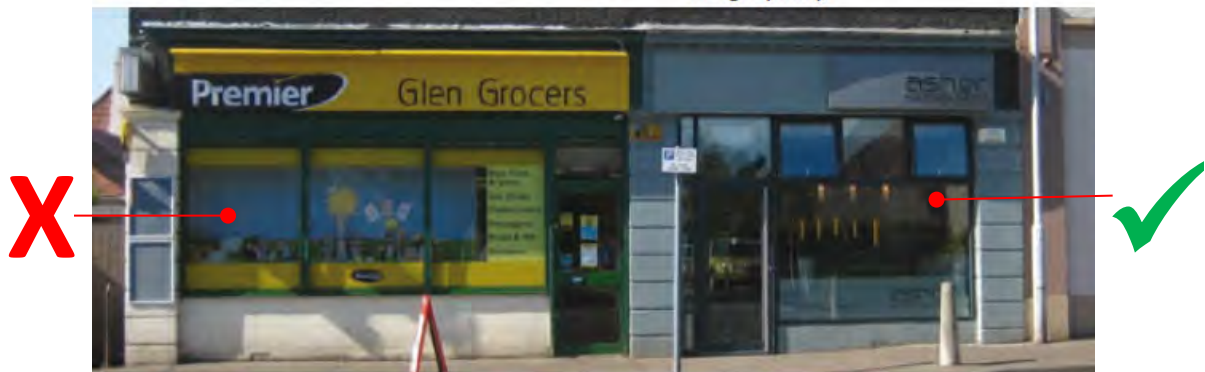
Above: Contrasting modern shop front treatments to similar adjoining units. The accumulation of relatively small differences to the unit on left resulting in poor overall design quality [source: Fife].
