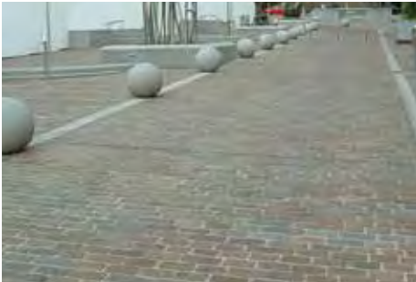
Natural stone paving used for shared surfaces
