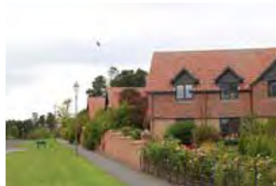
Fig. 3.55 Suburb housing at Wynyard Village County Durham
