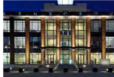
Uplighting to civic buildings
