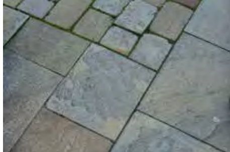
Traditional sandstone paving which is common to Lancashire
