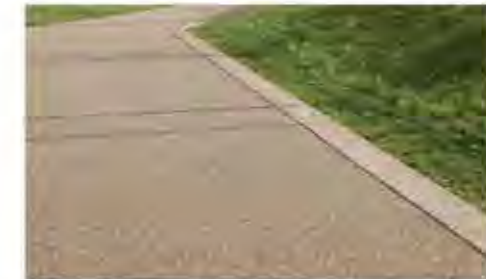
Resin bonded gravel path with edging
