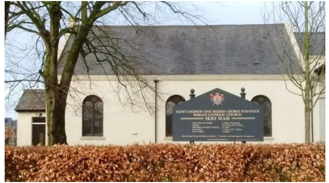
St Andrews and Blessed George Haydock Church
