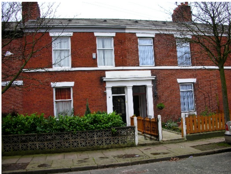
Figure 13: Principal elevation of 16 & 17 St. Ignatius Square (west side)
