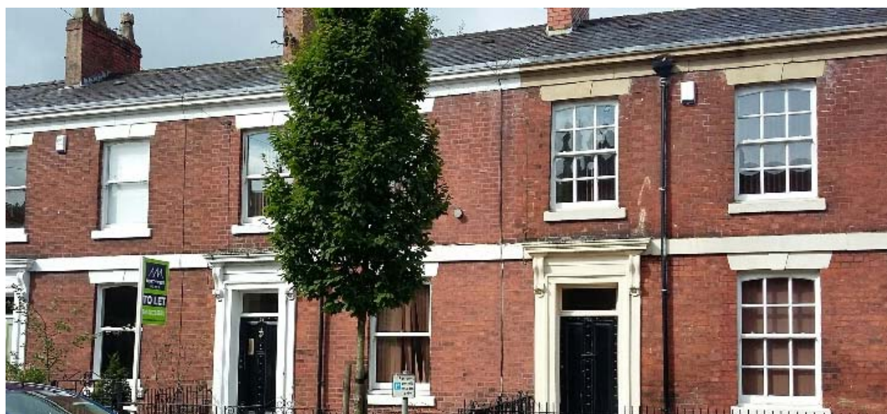
Figure 22: Variety of fenestration along St. Ignatius Square (west)
