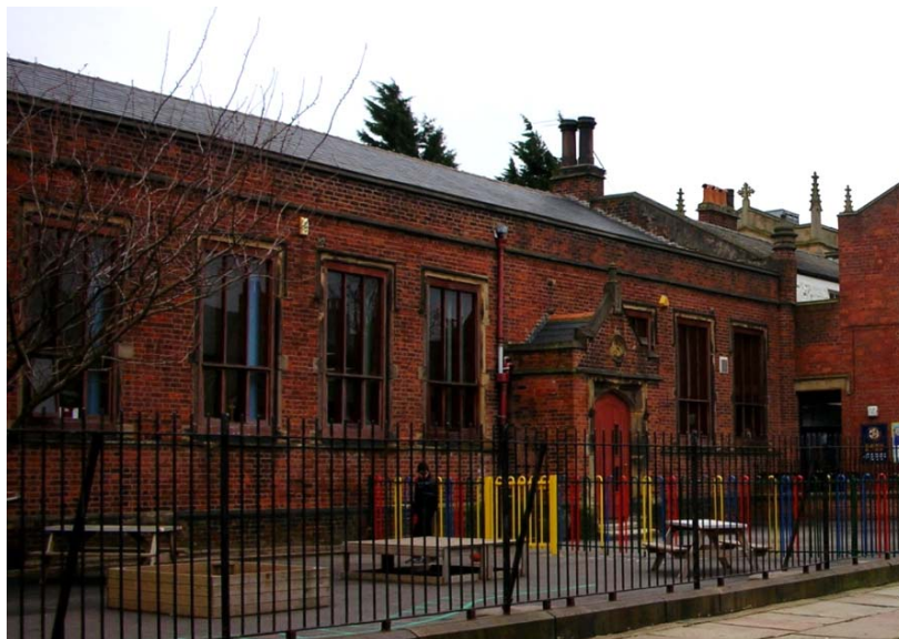
Figure 10: Western elevation of St. Ignatius School with the Church in the background
