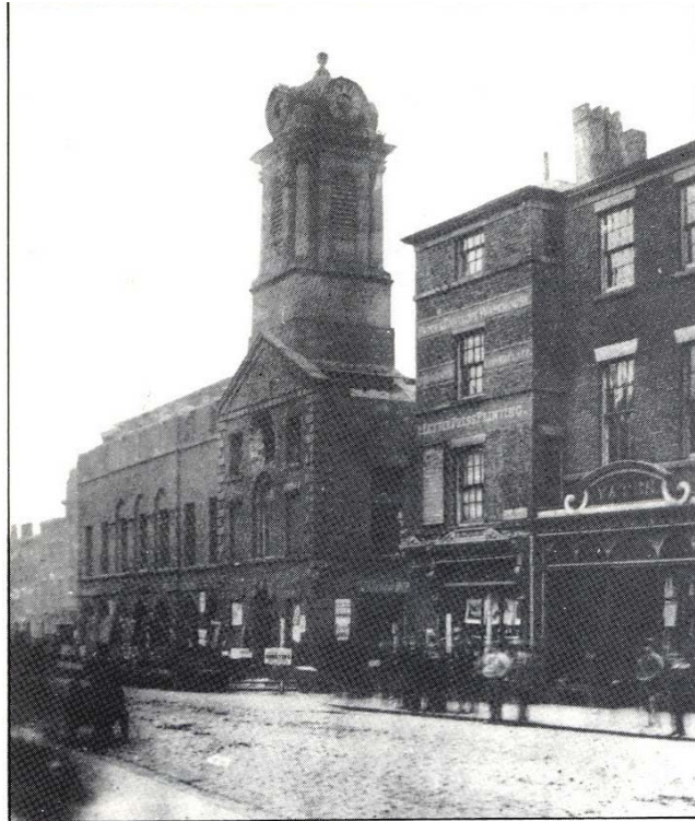
Fig 5 Photograph c. 1862 showing the Fishergate elevation of the Town Hall. On its left is the Guildhall and on its right are the buildings demolished to make way for the Miller Arcade.
