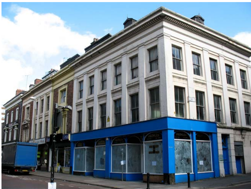
Fig 26 Stucco on some of the facades of Nos. 50 – 60, Lancaster Road
