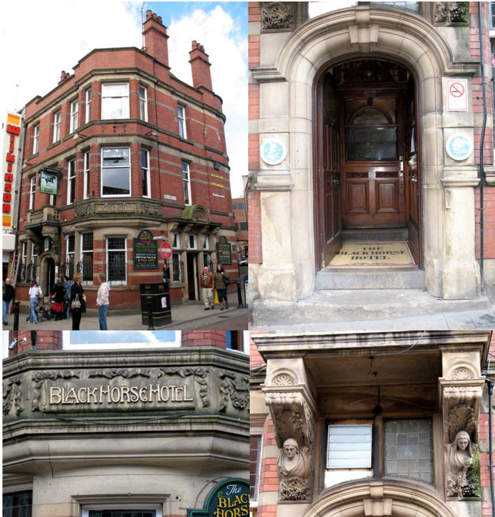
Fig 27 Clockwise from top left; the Black Horse seen from the corner of Orchard Street and Friargate, the main entrance, lettering above the door and the porch supported by caryatids
