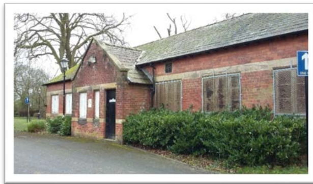
Figure 19 former laundry building, windows blocked up with security grilles and walls in need of re-pointing
