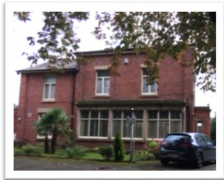
• Figure 30 15 Watling Street Road
