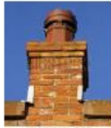
✓ WELL MAINTAINED CHIMNEY STACKS
