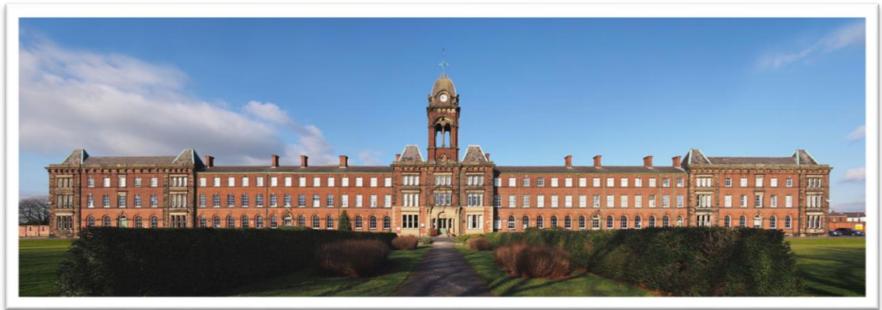
Figure 5 The former Preston Union Workhouse
