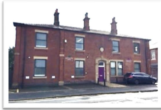
Figure 6 Former Police Station, Watling Street Road
