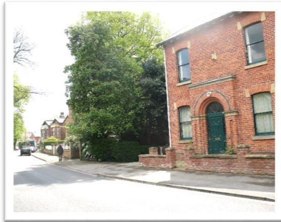
Figure 8 View east along Lower Bank road showing the curve of the road and a mid-18 th century detached house with original features
