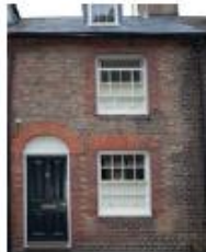
✓ TIMBER SLIDING SASH WINDOWS
