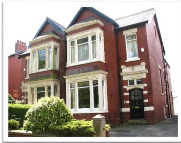
Figure 4 Typical examples of semi-detached properties on Watling Street Road
