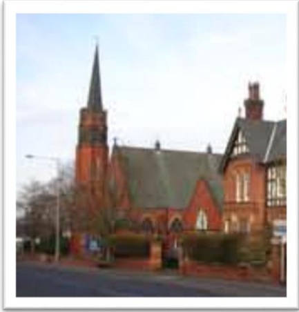
• Figure 28 Fulwood Methodist Church, Watling Street Road
