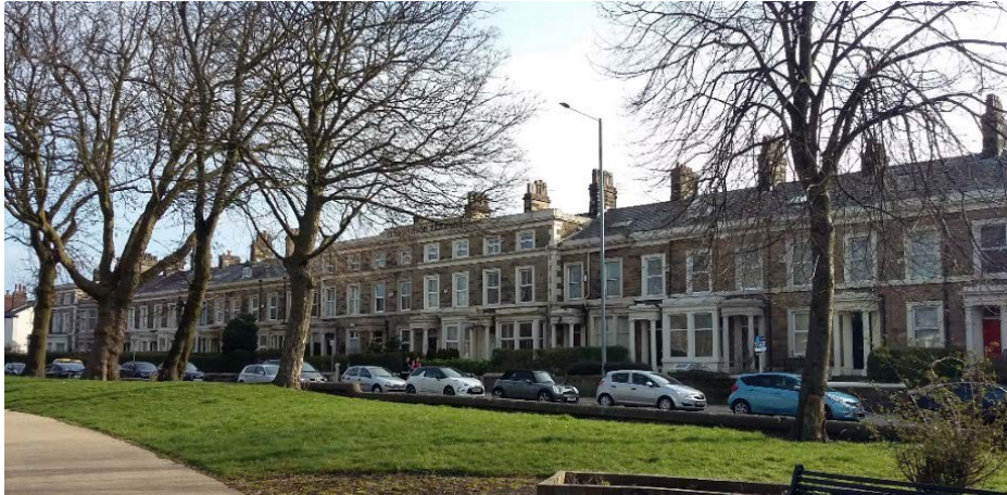
Figure 10: view of Stephenson Terrace looking north from within the park
