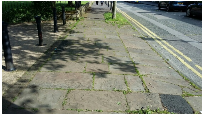
Figure 22: traditional stone flags to the park's entrance gates on East View
