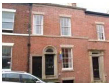
Six-over-six Sash Windows
