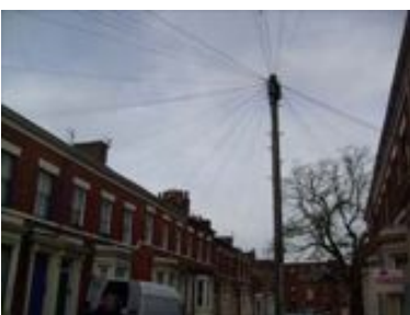
Telephone Wires on Bairstow Street
