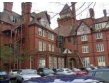
Former Railway Hotel
