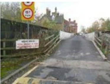
Modern Ramp Over Railway Bridge
