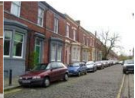
Bay Windows in Bairstow Street
