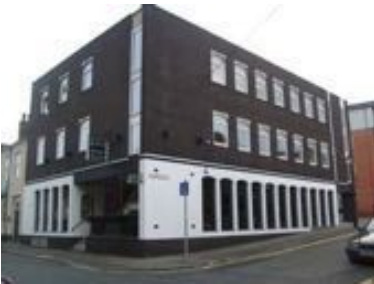
Intrusive Building on Chaddock Street
