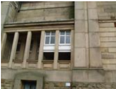
Intrusive Addition to Harris Institute
