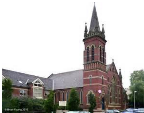
Ashton Methodist Church, Wellington Road
