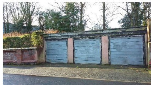
Flat roofed garages
