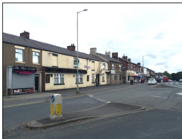
Vacant former public house on Longridge Road
