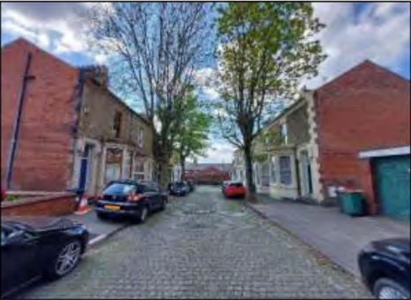
Setted street and pavement with stone flags on Cliff Street
