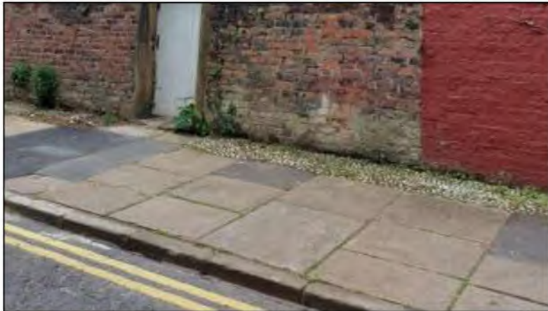
Example of stone pavement with cobbled strip; also note the repairs (left) on West Cliff Terrace and West Cliff
