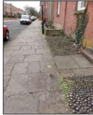
Example of stone pavement with cobbled strip; also note the repairs (left) on West Cliff Terrace and West Cliff
