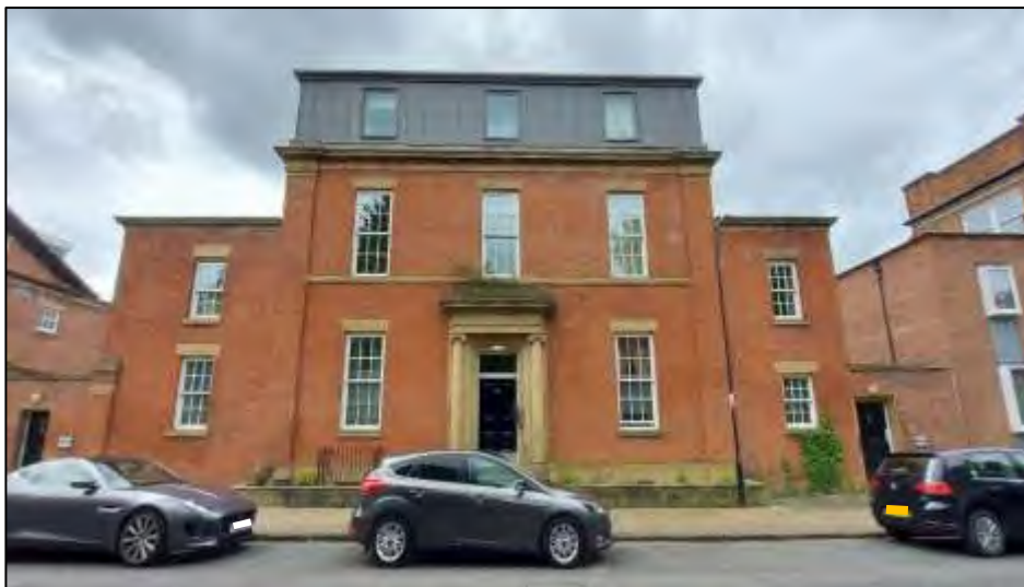
Roof extension of 48 West Cliff
