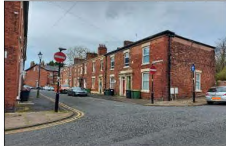
Four lampposts and attached signage result in a cluttered appearance on North Cliff Street
