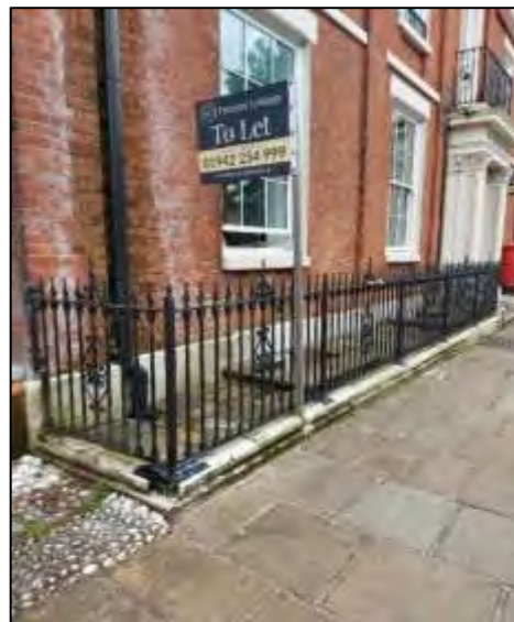
An example of replacement ironworks
