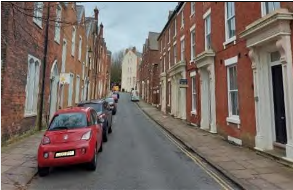
Stone flag pavement with tarmac street surface (Walton's Parade)
