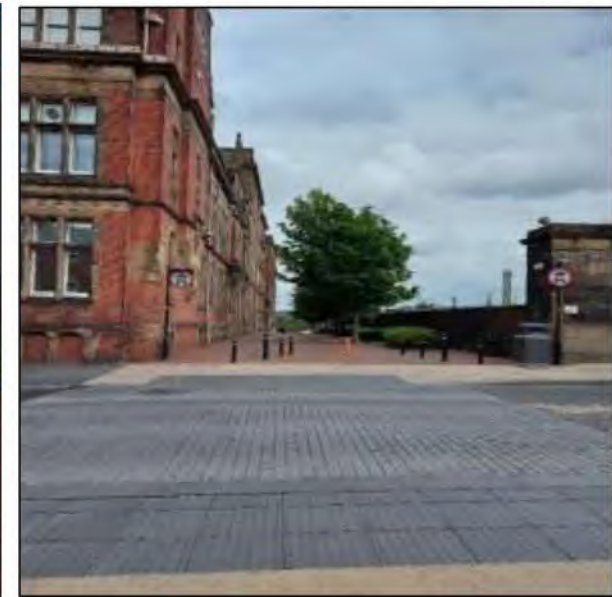
Block paving on an uncontrolled pedestrian crossing on Fishergate looking towards Pitt Street (note the variety of paving materials)
