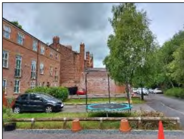
Knee rails located on West Cliff Terrace, highlighting the boundaries on the modern developments
