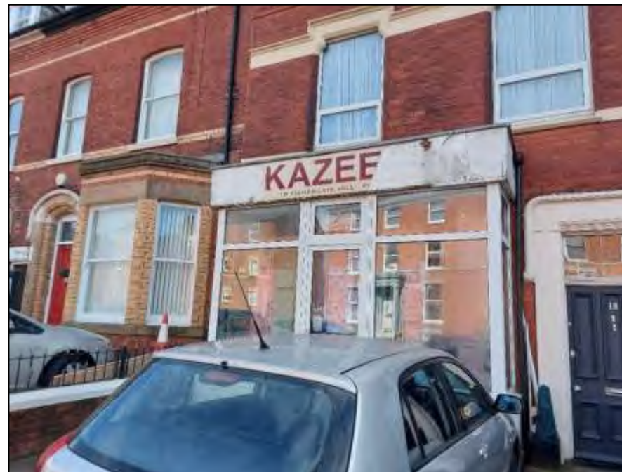
Poor shopfront design along Fishergate Hill
