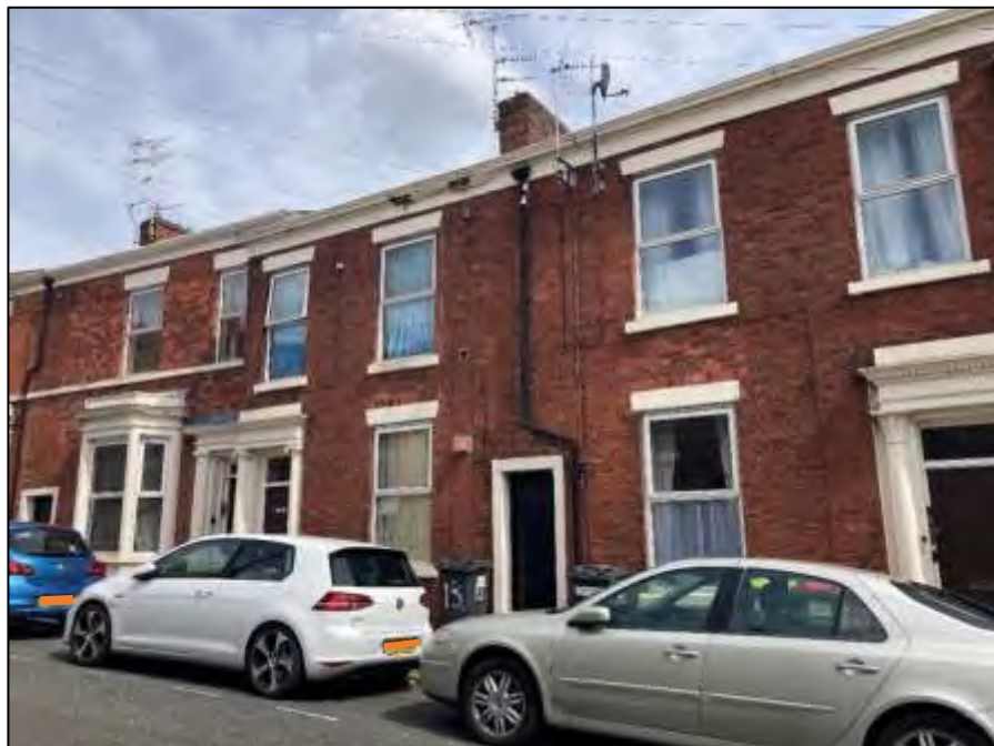
uPVC windows along Stanley Place
