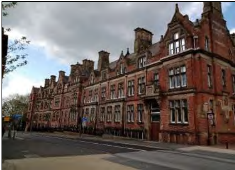
Iron railings mounted on stone bases at County Hall
