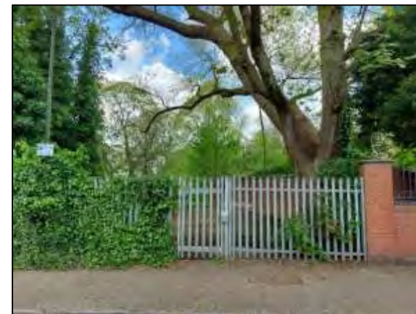
Palisade fencing and gate located at the north end of West Cliff
