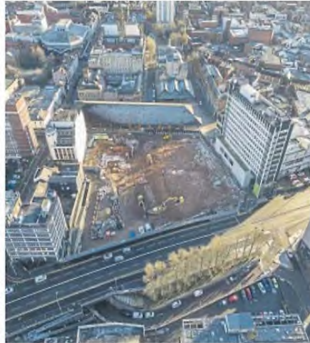
Eric Wright Construction started work on the site last month
