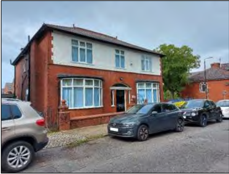
Interwar Terracotta boundary treatment on West Cliff, which are less common in the conservation area
