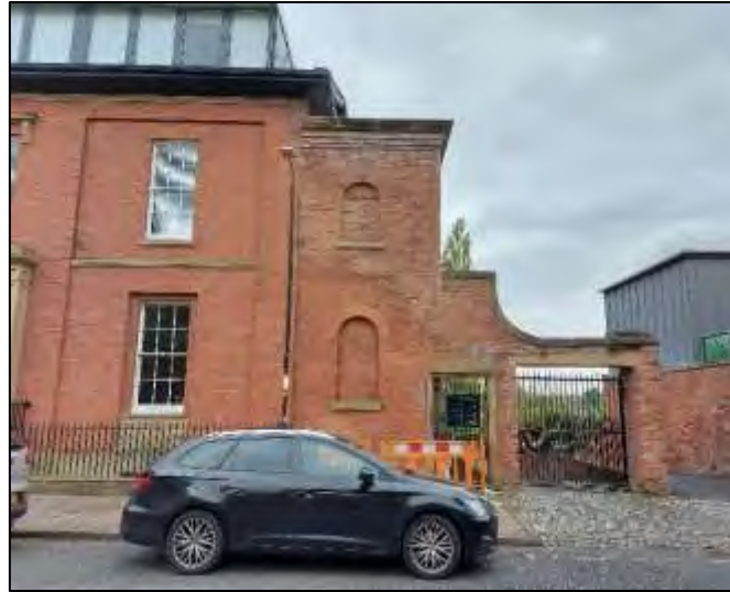
Ramped screen on West Cliff
