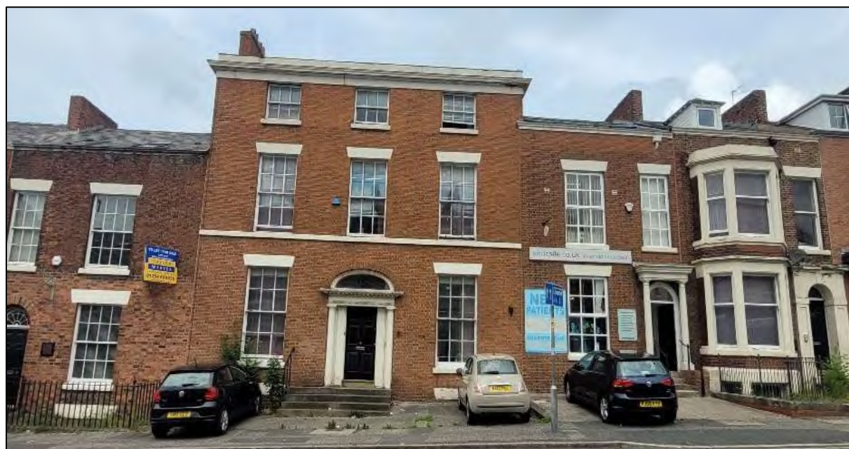
Properties on the north side of Fishergate Hill that have lost their gardens to off street parking.
