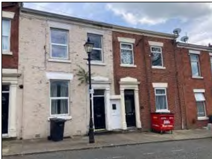
The introduction of a uPVC front entrance door between two properties
