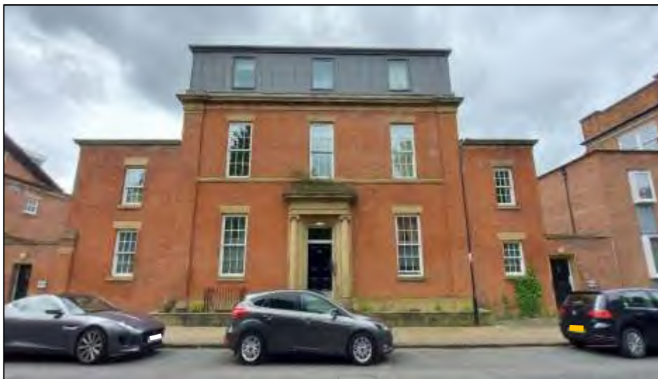
Roof extension of 48 West Cliff
