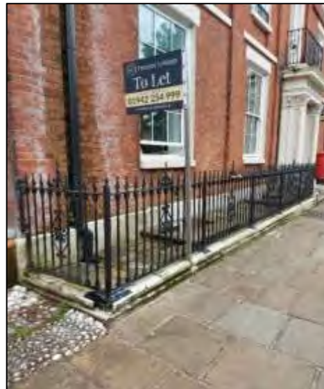
An example of replacement ironworks
