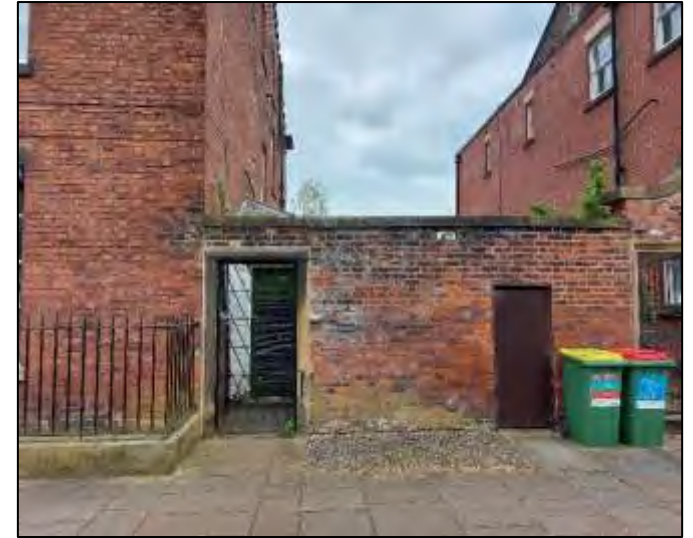
Tall boundary walls with gated entrances
