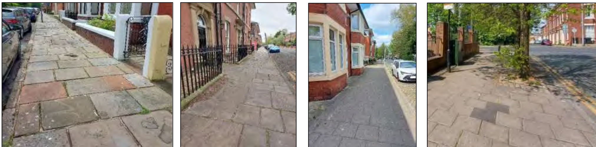
Example of stone flags with stone kerbs (West Cliff); Concrete flagstones on West Cliff, and tarmac infills on West Cliff (also note use of setts around trees)
