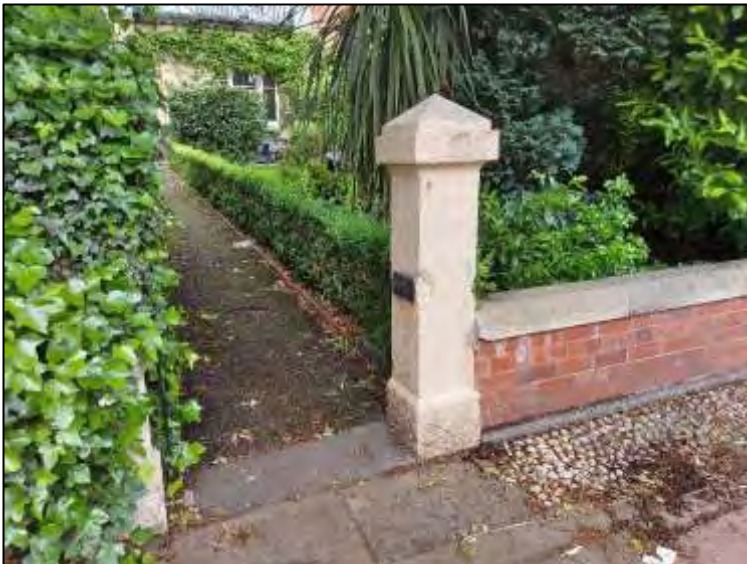
Brick dwarf walls with stone copings, a common boundary feature that would have originally had iron railings
