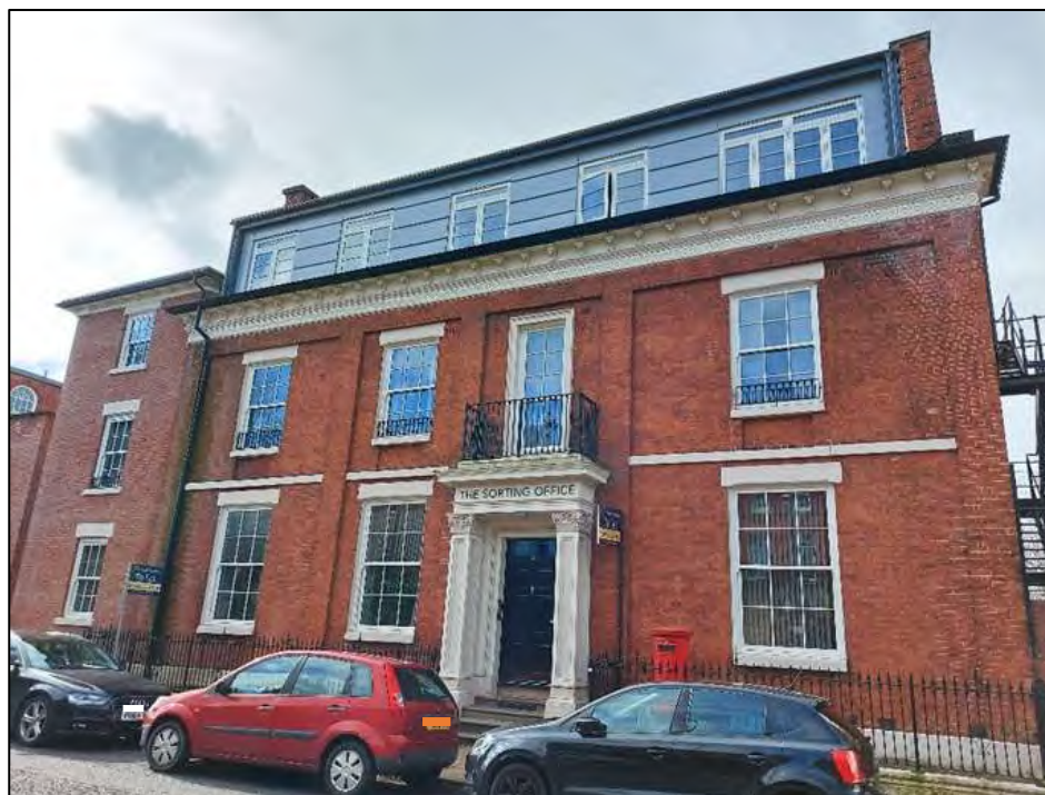
No.42 West Cliff after renovation work
