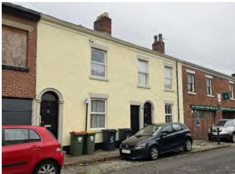
Rendered and painted brick elevations at 3-5 Great Avenham Street
