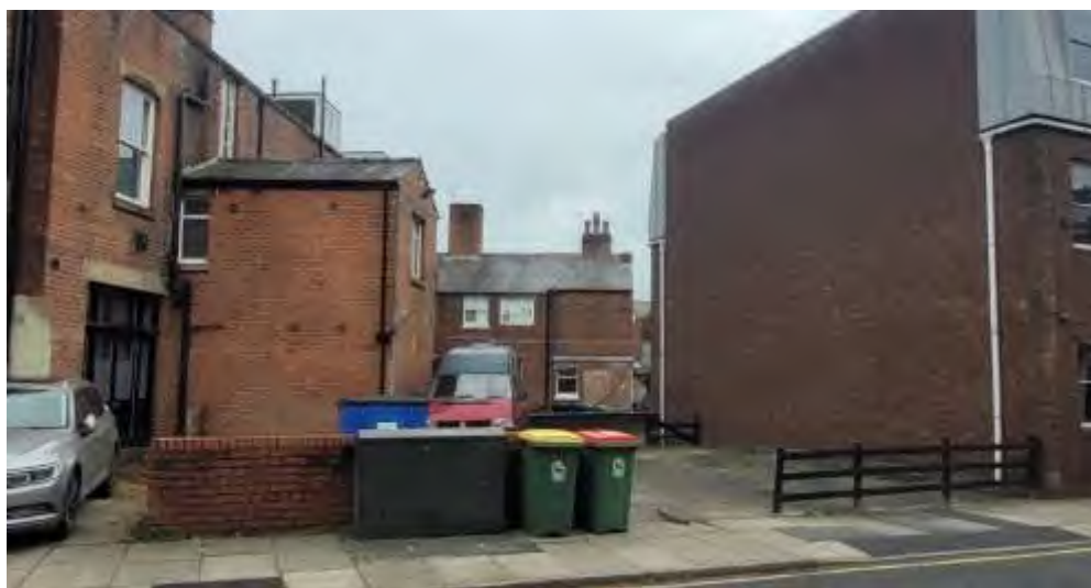
Rear garden of 29a Ribblesdale Place with hardstanding and mix of boundary treatments
