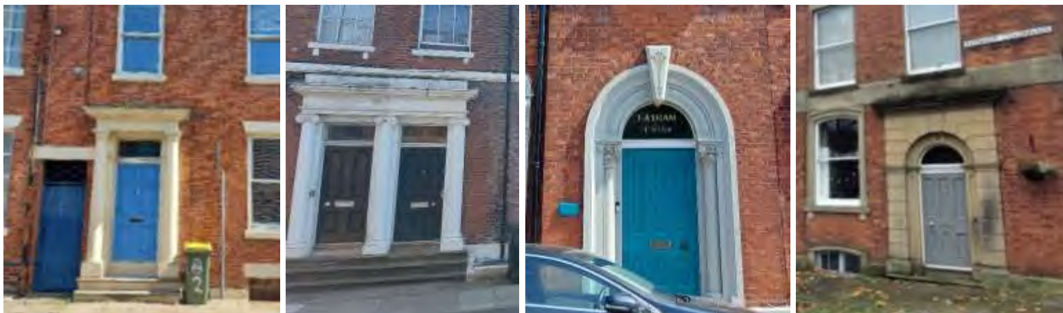
Examples of doorways in the conservation area
