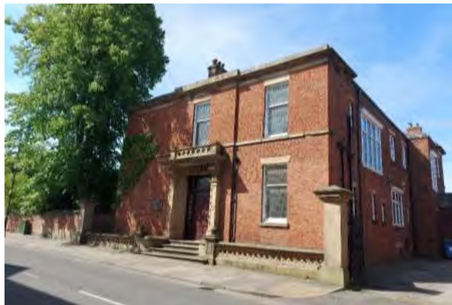
Boundary walls of 14 Ribblesdale Place
