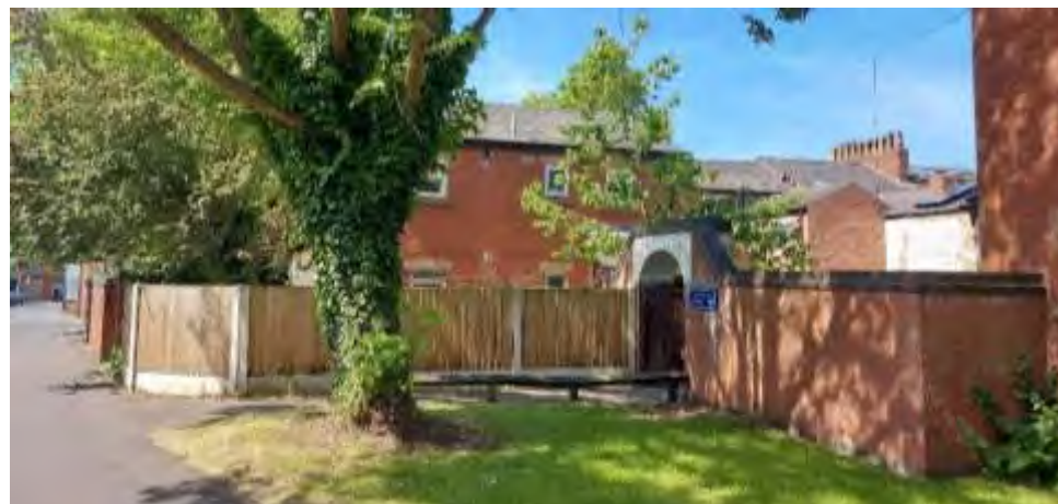
19 Avenham Lane timber boundary treatment
