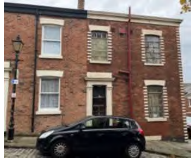
Alternating bricks, 57 Great Avenham Street
