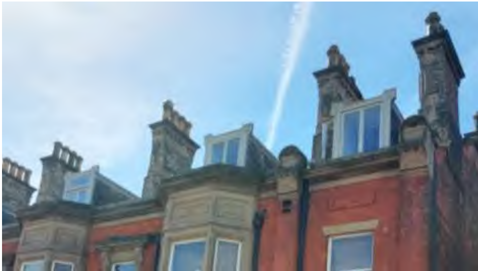
Chimney stacks, 6-7 Ribblesdale Place
