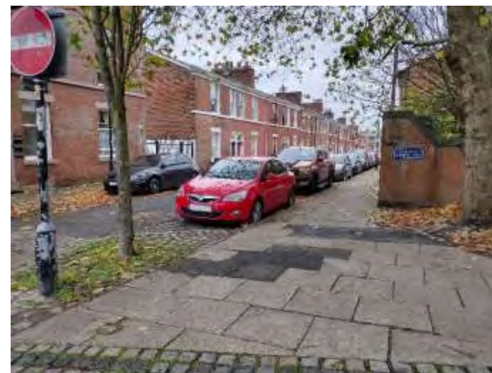
Repairs to flagstones along Chaddock Street
