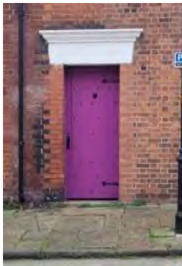
8 Regent Street through-lobby doorway with cornice and purple painted door
