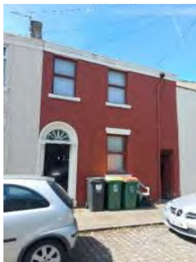
Painted brickwork; rendered elevation in poor condition
