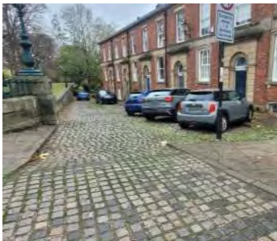
Stone setts along Avenham Colonnade
