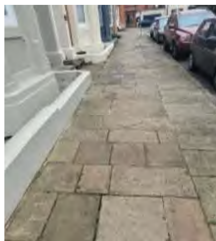
Stone flags along Camden Place
