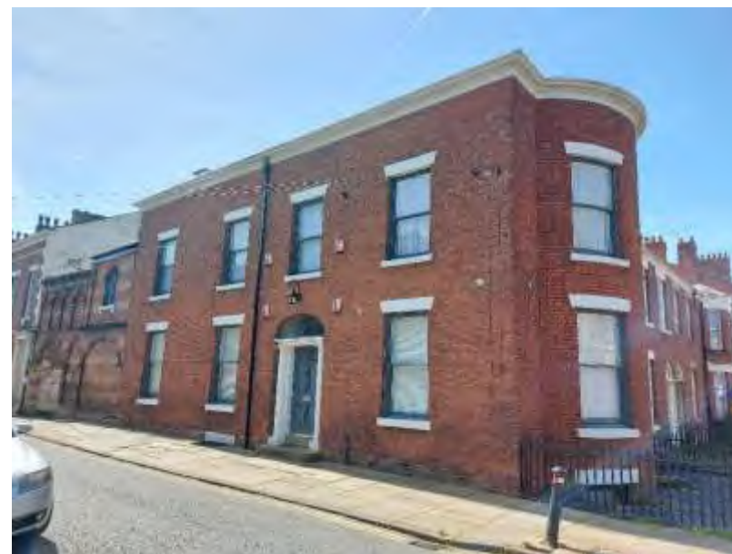
Bow window, 29 Latham Street
