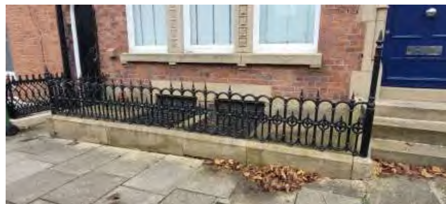
Railings 6a Starkie Street
