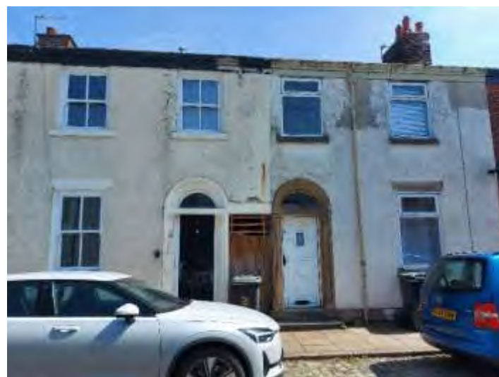
Painted brickwork; rendered elevation in poor condition
