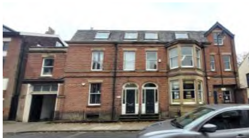
Rooflights at 10-11 Ribblesdale Place
