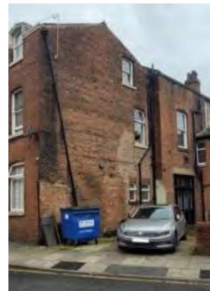
Brick repairs and traces of the removed boundary wall
