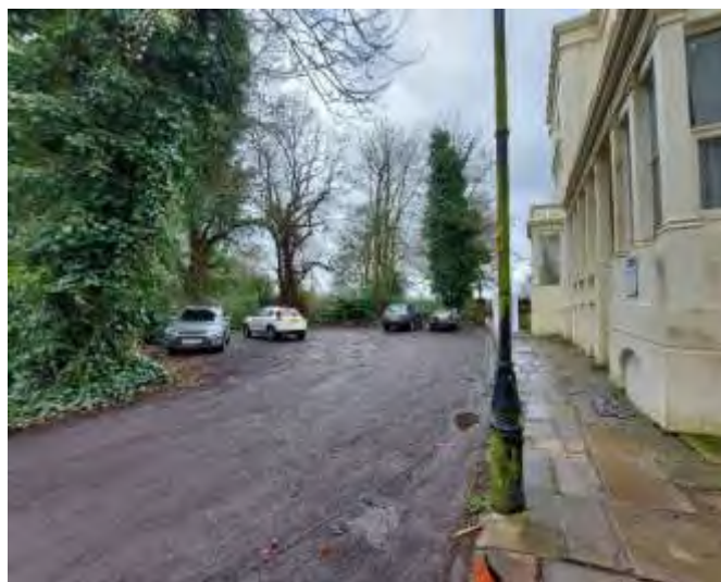
Bank Parade road surface
