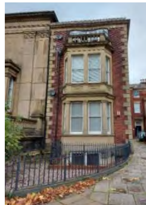
38 Bairstow Street iron railings
