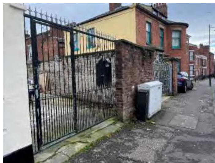
Tarmac footpath along Avenham Lane
