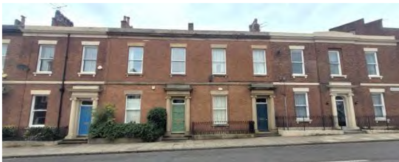
Doorways with Ionic columns and six-panelled doors at 30-34 Ribblesdale Place
