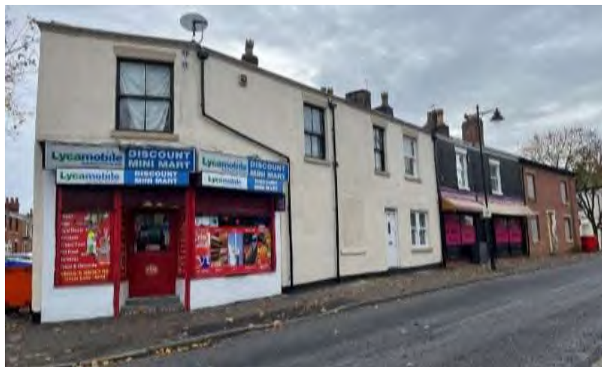
24-32 Avenham Lane with shops (left end and black painted house) and vacant pub (right end)
