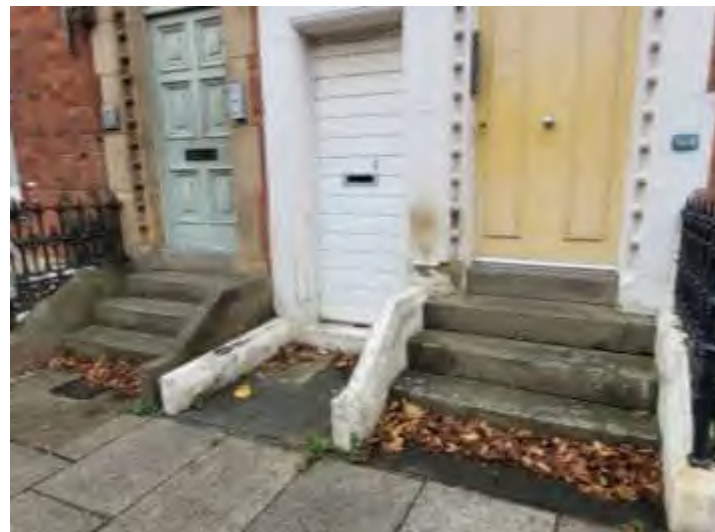
Altered through-lobby door between 7 and 8 Starkie Street
