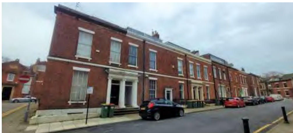
Dormer windows 3-6 Starkie Street
