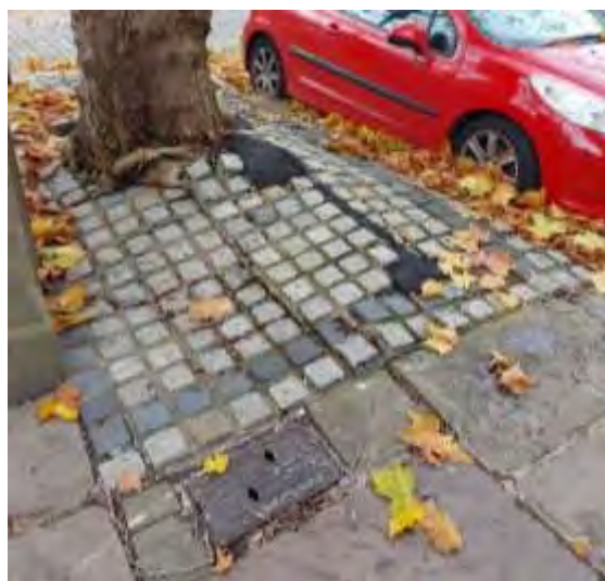
Repairs to setted area around tree on Bairstow Street
