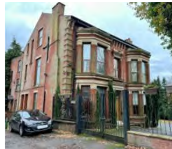
Brown uPVC windows of Oak House
