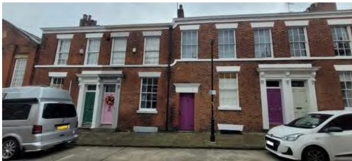
Traditional six over six timber sash windows on the northern end of Regent Street with door panels painted in a variety of colours
